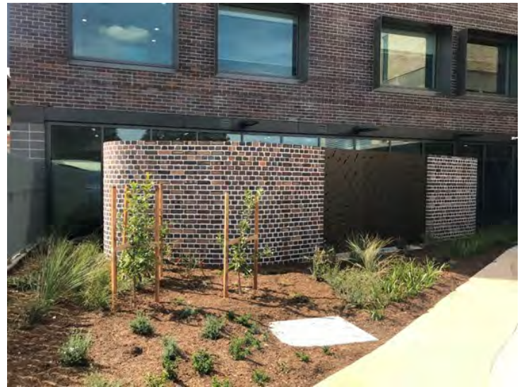
Emergency department entrance
