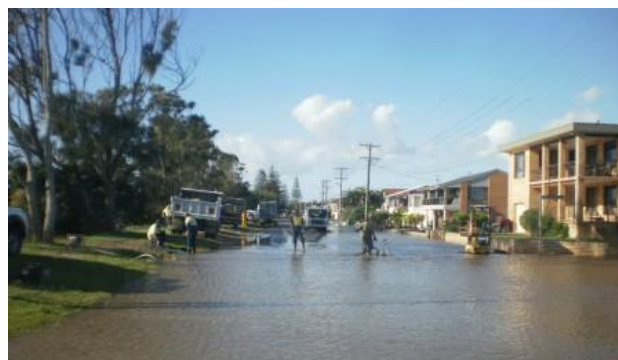
Maintenance to sewerage during floods
